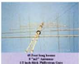
Fig. 5: Another antenna picture from Fred VE7PL's sit. The wording along the bottom reads: "45 Foot long booms, 8 "m2" Antennas, 0.5in thick Phillystran Guys".
